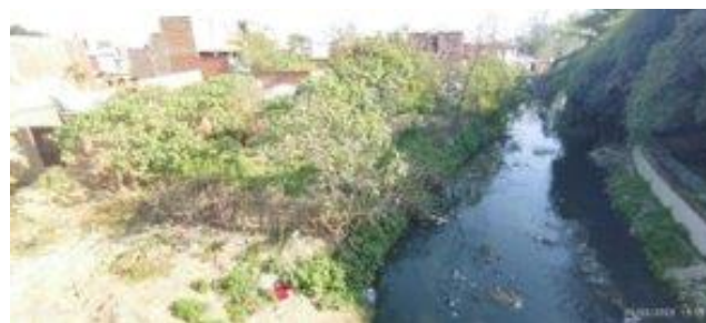
Figure 40 Encroached stretch sections: Nakatiya river
