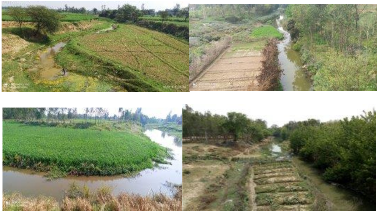
Figure 41 Encroached stretch sections: Aril River
