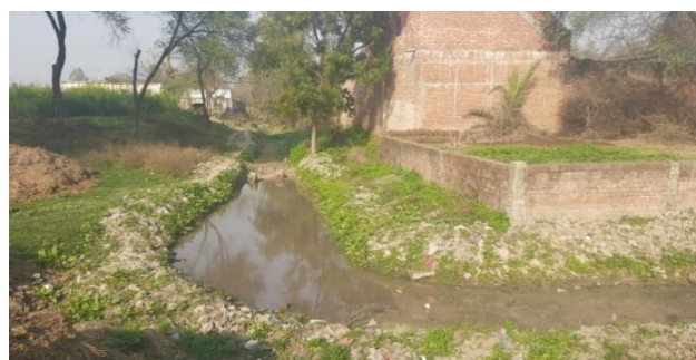
Figure 42 Encroachment and choking of wetland inlet (before and after rehabilitation)
